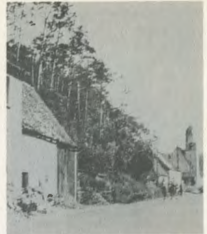
View south along Philippsbourg main street from below Main Forks. The considerable distance to the Lutheran church from Main Forks is evident. Snapshot taken in summer of 1945.
