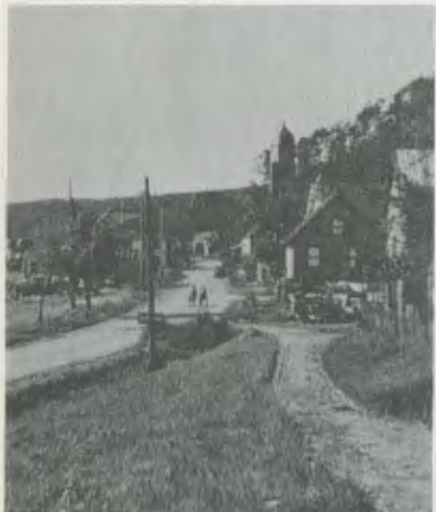
View into Philippsbourg from the south shows main street almost up to Main Forks. Rock formation faintly visible on the skyline is on the ridge north of the village—274th A Co's objective on 5 Jan 45.
